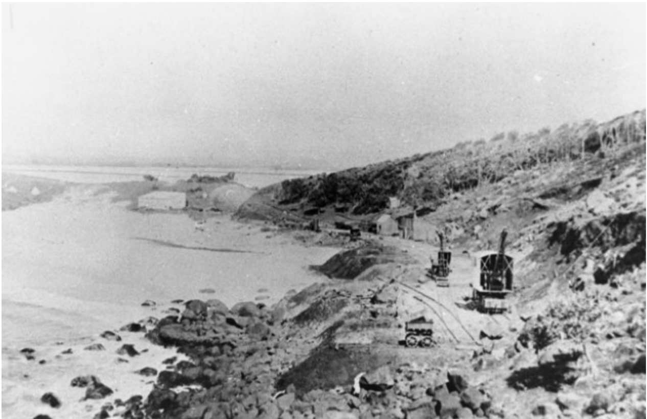
Figure 2 Quarrying of Point Danger basalt in order to build the original Tweed River training walls, circa 1890 -1910 (Guthrie, 2011)
