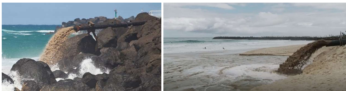
Figure 28 Sand pumping at Duranbah Beach; (left) off the northern training wall (source: Joli). (right) via temporary pipeline to the northern end of Duranbah Beach (source: Coastalwatch)
